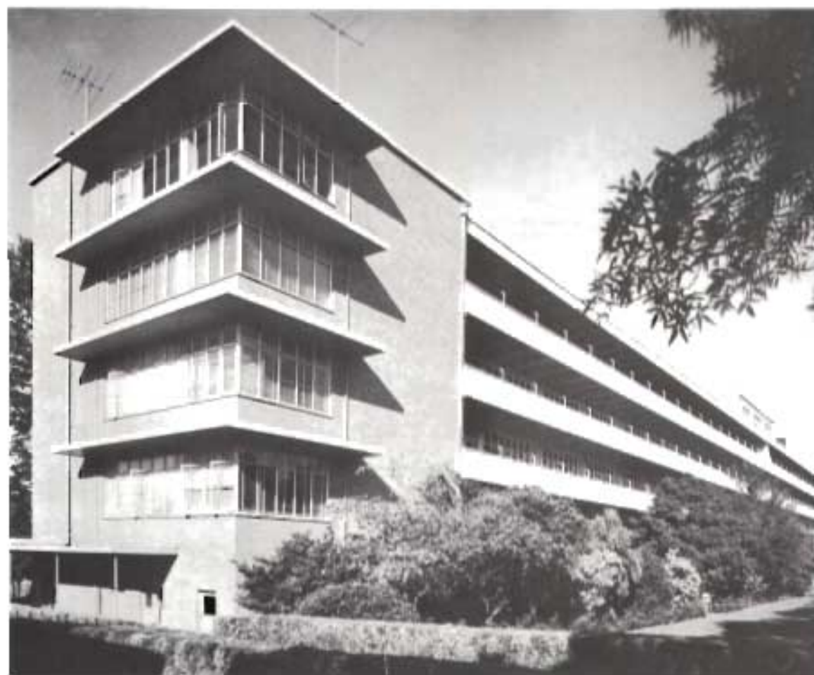
The main block of the Repatriation General Hospital, Heidelberg. Repatriation Department
