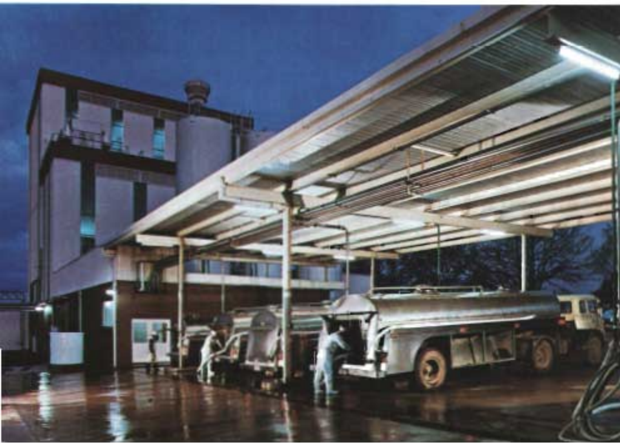
Bulk carriage terminal for milk. Australian Dairy Producers Board
