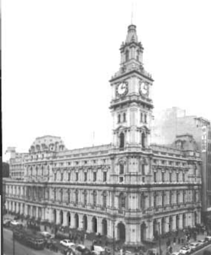
The General Post Office, Melbourne, which is also shown in the photograph below.
