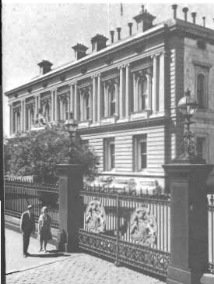
The former Royal Mint, now used for performing civil marriages.
