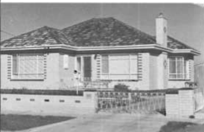
A triple fronted brick veneer house, typical of many built in the 1950s and 1960s.
